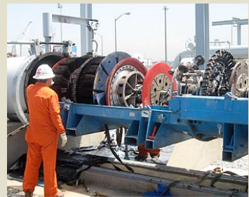
A "smart pig" being readied for an internal pipeline inspection
